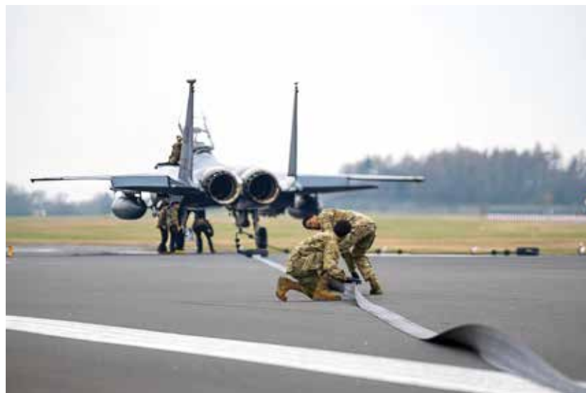
A MAAS was installed and certified for the first time on RAF Fairford in support of Ramstein Flag 2025 providing critical safety and operational capabilities for participating NATO forces. Photo by Jessica Avallone
