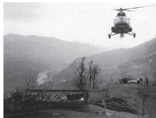
In the years of the People's Republic of Romania, helicopters were used also in the economy. The images show Mi-8 helicopters working for the installation of high-voltage poles in mountainous areas (above) and for the construction of a power plant funnel (below)
