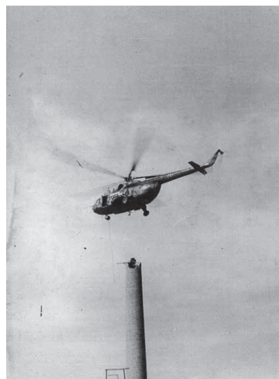
In the years of the People's Republic of Romania, helicopters were used also in the economy. The images show Mi-8 helicopters working for the installation of high-voltage poles in mountainous areas (above) and for the construction of a power plant funnel (below)
