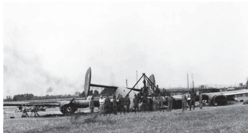
Romanian military and perhaps civilian personnel take a moment pose for a picture during the salvage of the wreck of the B-24D "Brewery Wagon." One can get an idea of the size of the aircraft from its 110-foot wingspan. The men have erected a hoist near the flattened forward end of the bomber, with the only thing to stop the complete crushing being the aircraft's four engines. Note what appears to be a pair of jacks under the wing at the left, which are actually two rifle stacks of the soldiers working at the site. Some industrial facilities on the edge of Ploiesti are seen in the background. Most of the major components of the many downed B-24 bombers were scrapped, though some still-useable parts were repurposed for other things.
